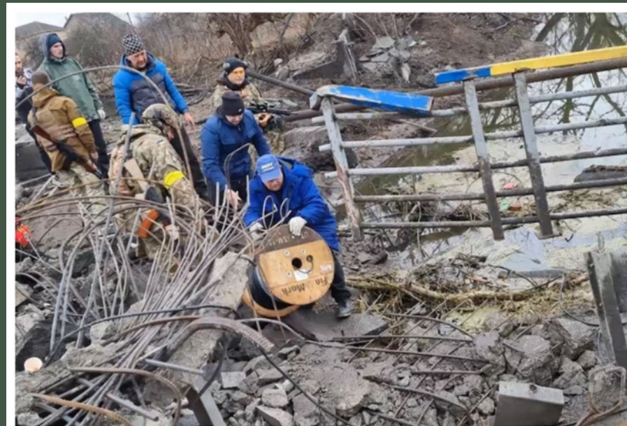
An internet network repair crew rolls out cable to restore connectivity in the city of Irpin, near Kyiv. (Supplied: Yuriy Matsyk)
